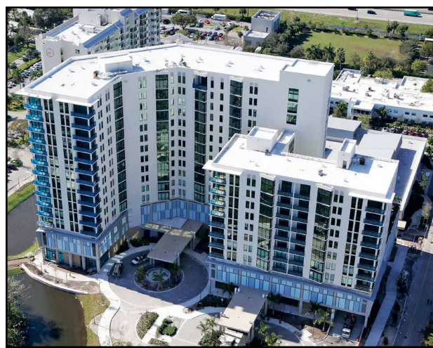
The first moves begin this month into Westlake at JKV.
