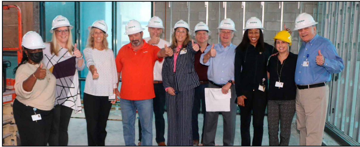
The JKV Management Team tours the construction inside The Vue and The Terrace at Westlake.
