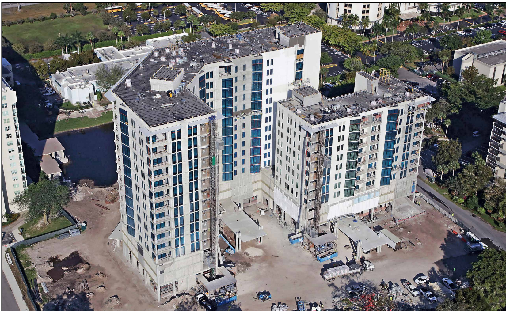
The 15-story Vue and 11-story Terrace are now undergoing interior finishing and installations.
