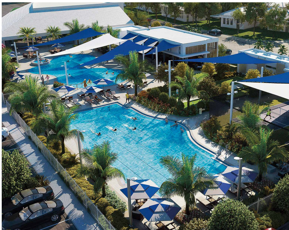
The John Knox Village Aquatic Complex is nearing completion.
