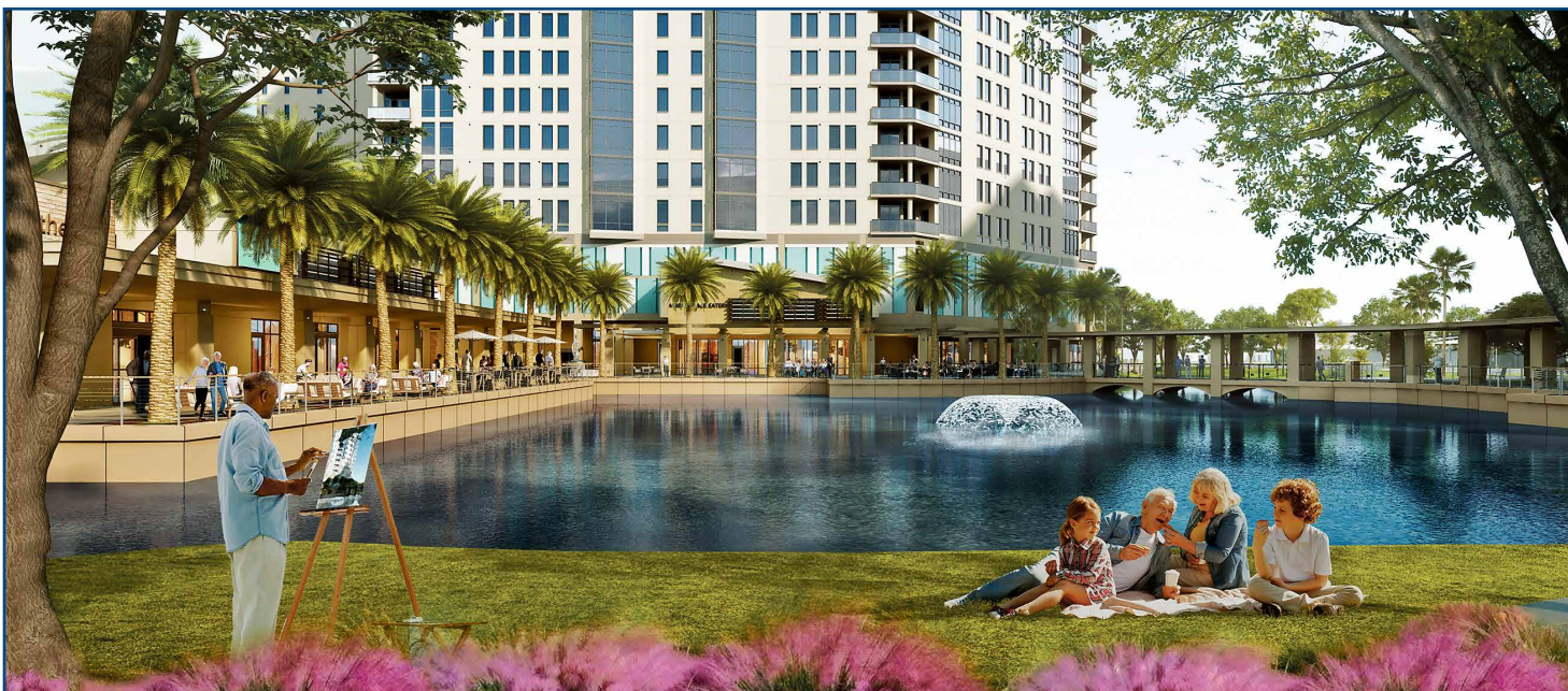
Construction of the Westlake Pavilion is on schedule for a first quarter 2022 opening at John Knox Village.
