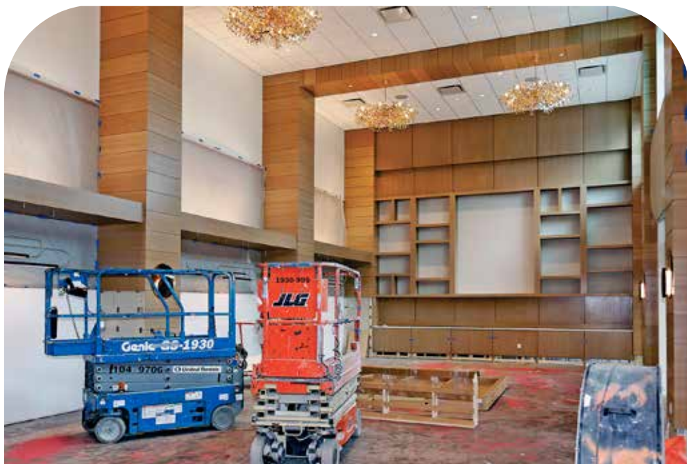
Crews are finishing construction inside the Pavilion and the Seaglass restaurant.
