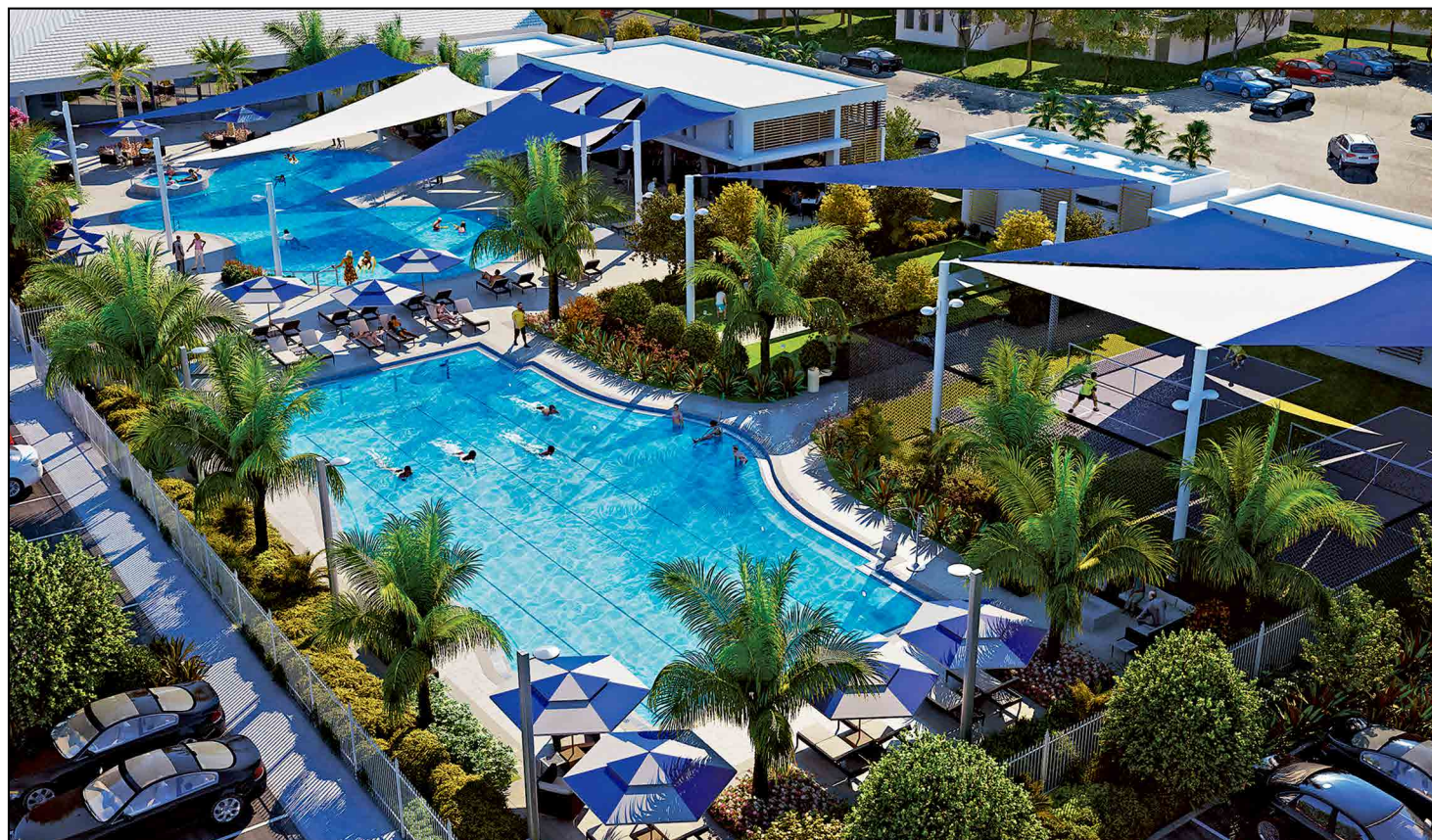
The new Aquatic Complex is now under construction. When completed the complex will feature a walk-in zero-entry resort style pool, a four-lane 25-meter-long lap pool, 60-seat indoor restaurant, an open-air sports bar and grille, two each pickleball and bocce ball courts, a Jacuzzi and fire pit.
