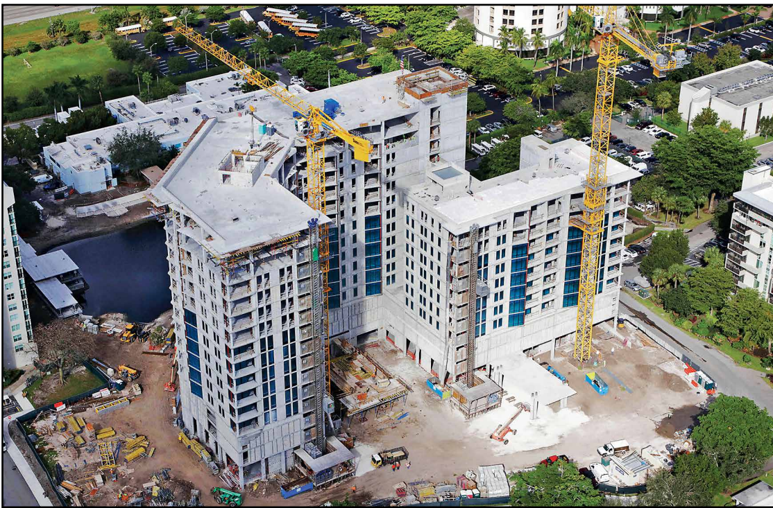
The 11-story Terrace (foreground right) and 15-story Vue apartment buildings have topped out and are entering the interior finishing phase of construction.
