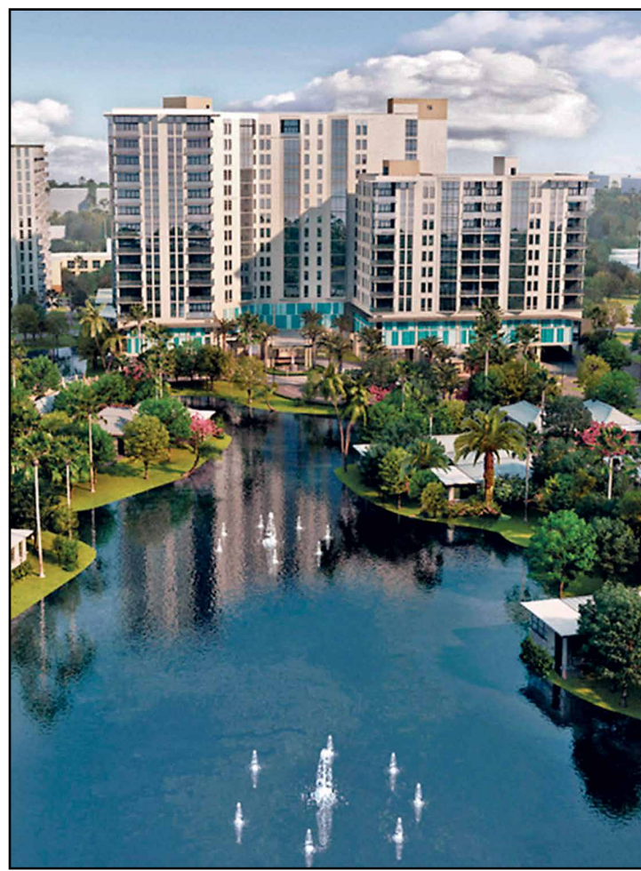
Construction has begun on the two new Westlake apartment buildings: The Terrace and The Vue.
