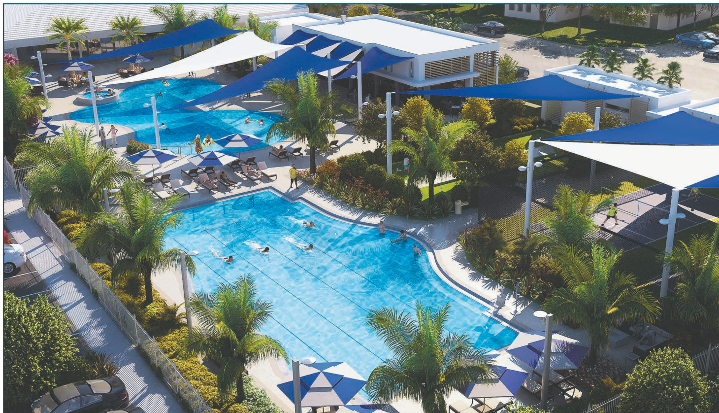
When completed later this year, the Aquatic Complex will include a resort-style pool, a four-lane 75-foot long lap pool, a 60-seat Tropics Grille indoor restaurant, an open-air sports bar, two each Pickleball and bocce ball courts, a Jacuzzi and fire pit.
